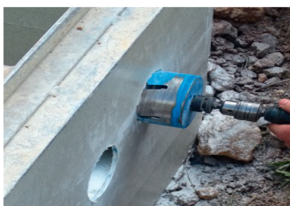
4. Use a hole saw to cut the connections for the empty conduits into the wall of the cable distribution box at the appropriate positions. The base and head spacer frame must not be drilled through.
