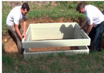
2. Position and align the first pre-mounted spacer frame as a base with mounted floor. Mount each additional spacer frame and latch it evenly to the lower spacer frame.
