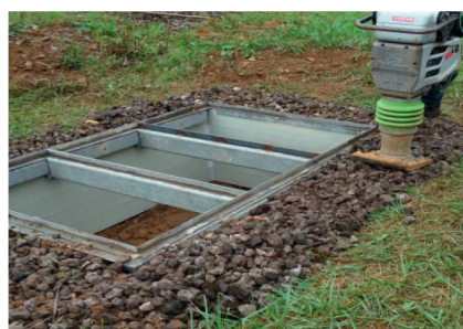
5. Fill the excavation flush to the top edge of the steel frame and compact with a vibratory rammer.
