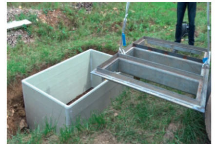
3. The top is formed by the head spacer frame with pre-mounted steel frame. Position the top over the entire surface of the last spacer frame using a suitable lifting device and latch it in place.
