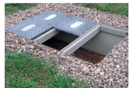
6. The GRP cover plates are inserted into the frame using a cover lifter.
